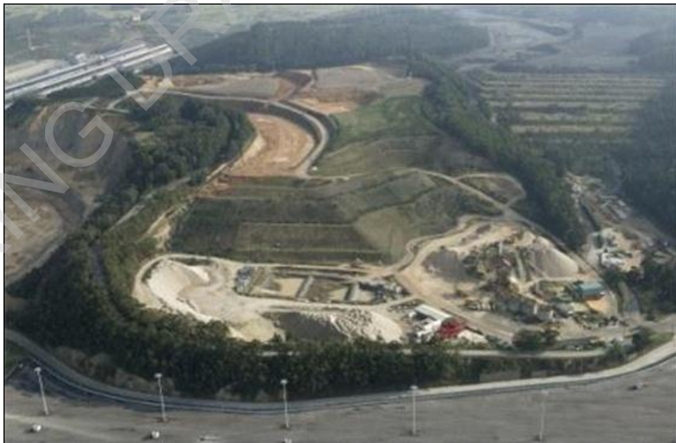
November 2011: landscape restoration ongoing with Jarofix
